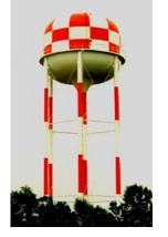
At any given time, the flow from the source may not be sufficient to meet the demand of the consumer. Because of this, a PWS utilizes water storage tanks. Water tanks are connected to the distribution system. These tanks will vary in both size and design. The tanks main purpose is to help maintain adequate flow to the consumer during peak demand hours.
