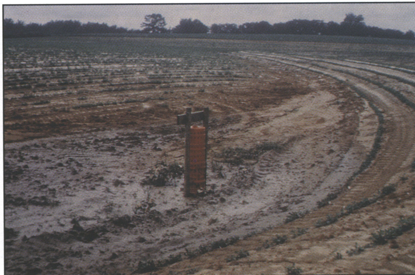
As runoff water pools in this basin, sediment is deposited and the water is slowly discharged to an underground pipe.
