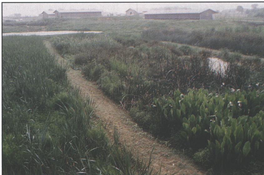
Wetland plants provide a high level of treatment for the effluent from a swine lagoon.
