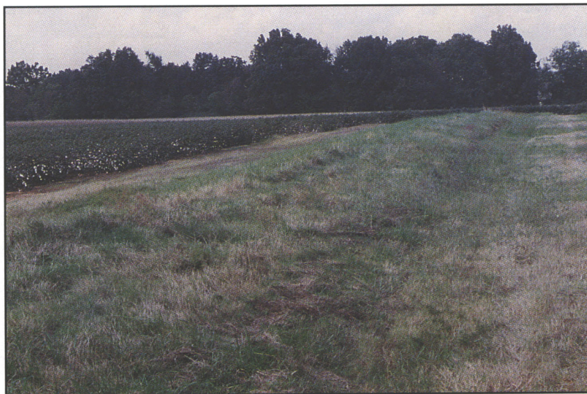
A diversion intercepts storm water and carries it across slope to a safe disposal area.
