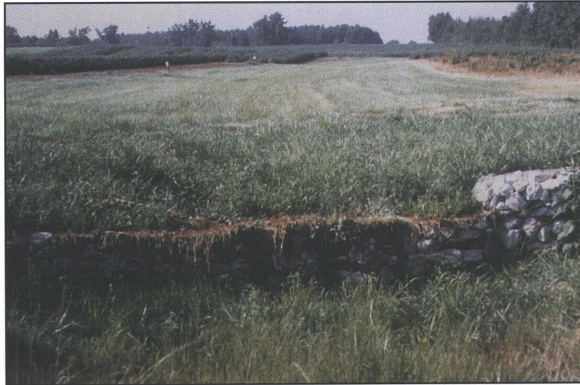
This structure is used to safely drop the flow of water from one elevation to a lower elevation without causing gully erosion.
