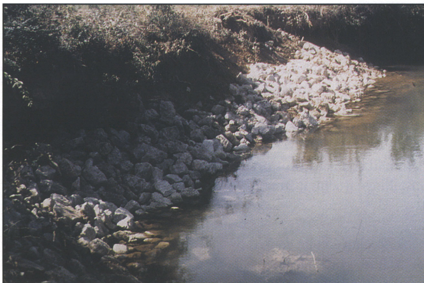
Rock riprap is used here to prevent scouring of the streambank.
