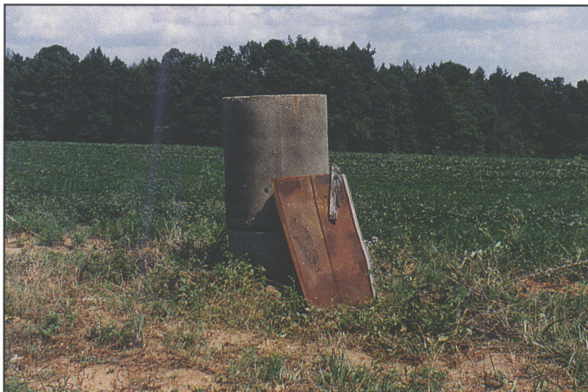
An unsealed abandoned well can be a safety hazard as well as a source of ground water pollution.
