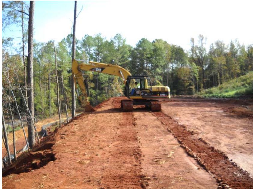
EPA reinforcing the lagoon banks
