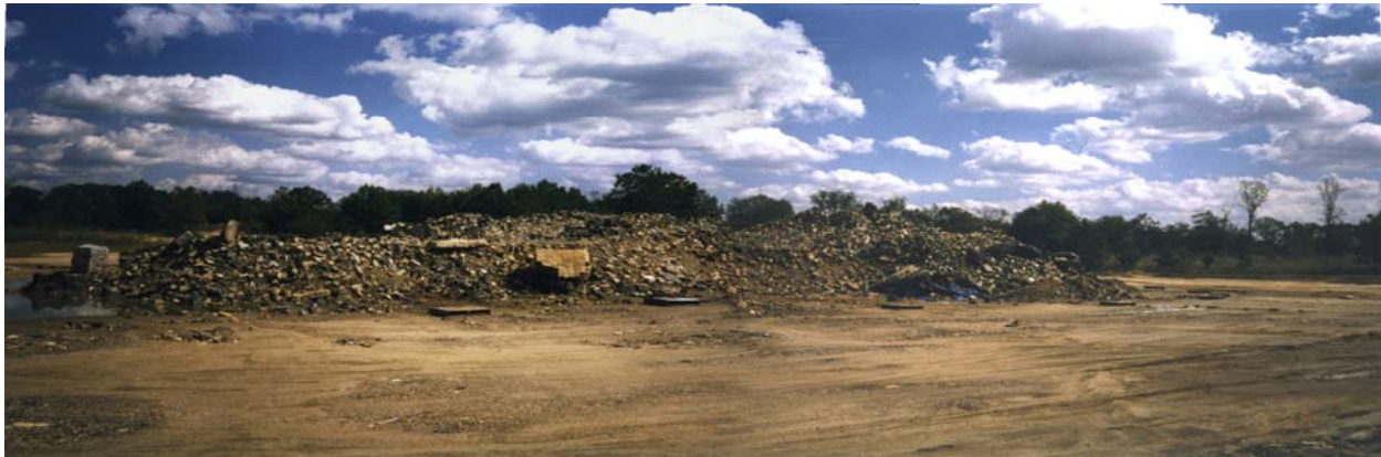
Foundry brick staged for removal
