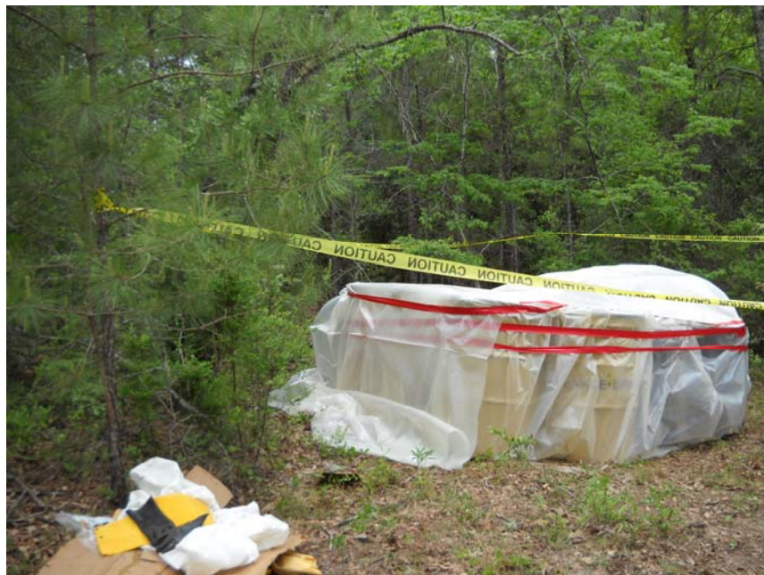
Drums and totes secured and ready for transport off-site
