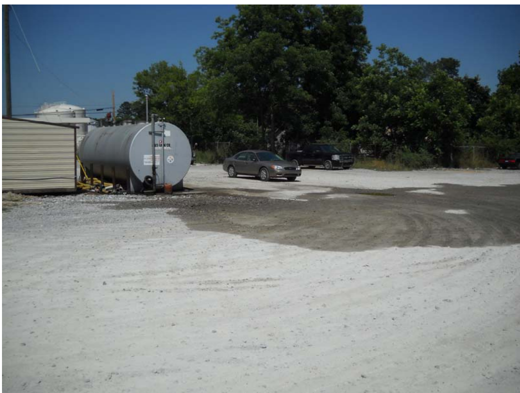
Above-ground diesel tank and leaked fuel
