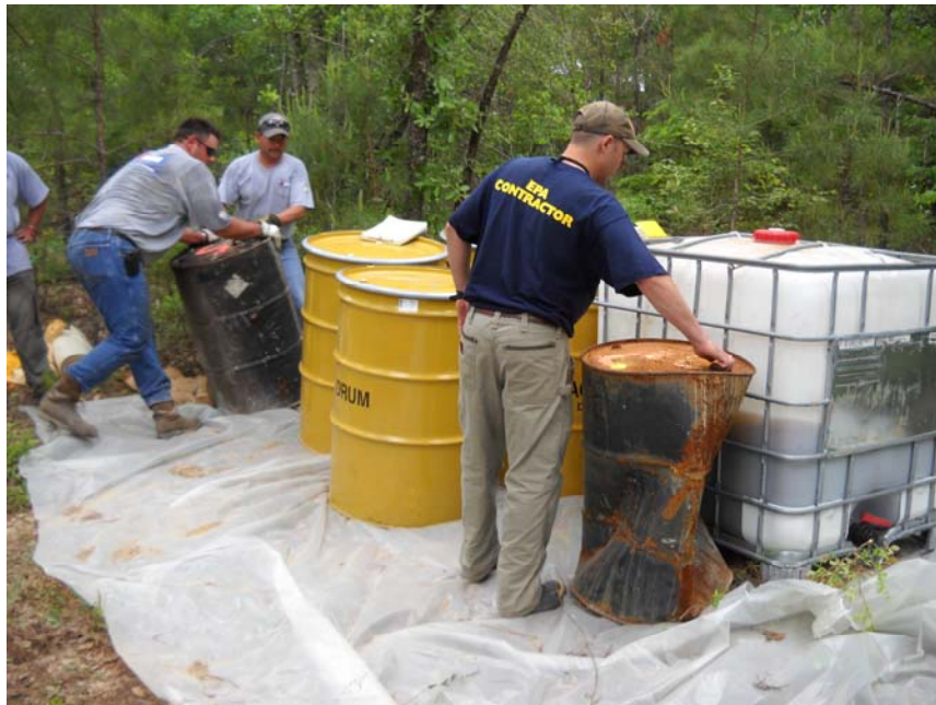
EPA contractors over-packing and staging drums and totes
