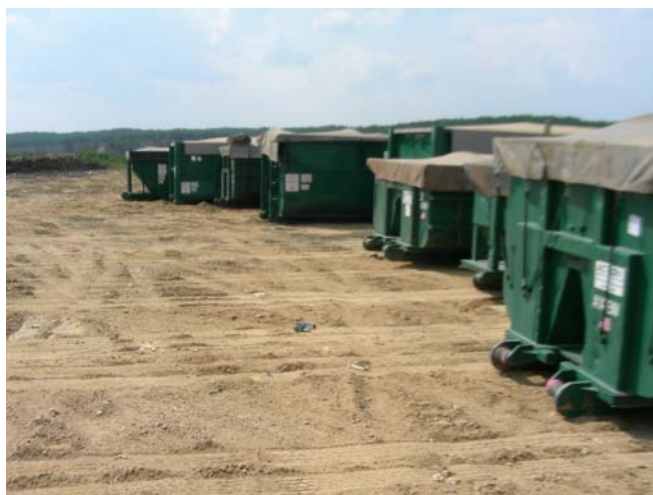
Roll-offs containing hazardous soil staged at the local landfill
