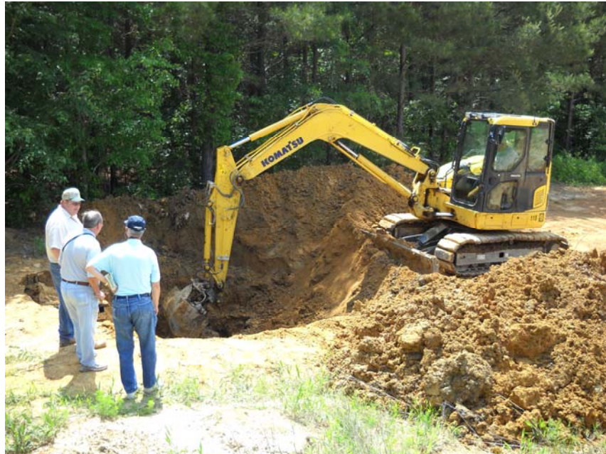
Excavation of burial pit on Cullman Road Department property
