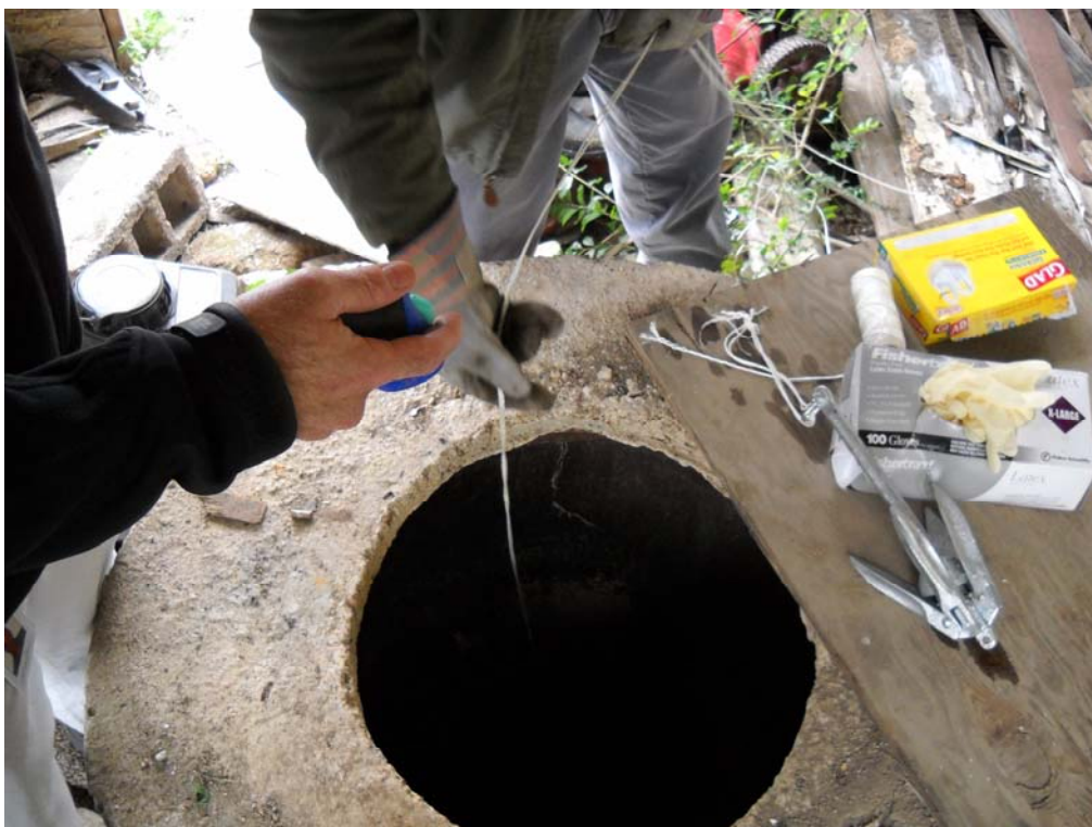
ADEM personnel inspecting and sampling the well
