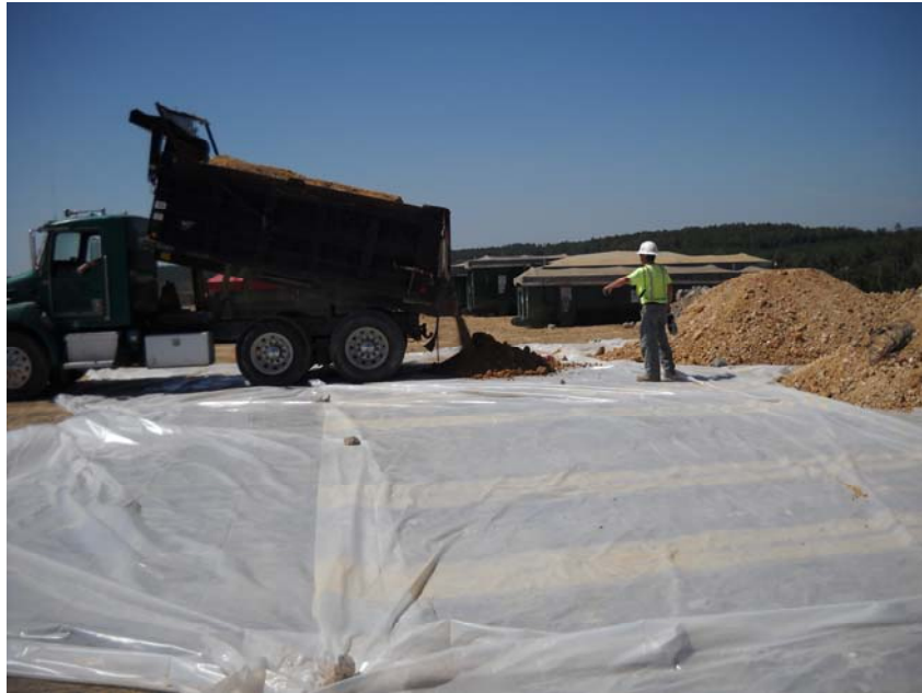
Non-hazardous surface soil removed from right-of-way
