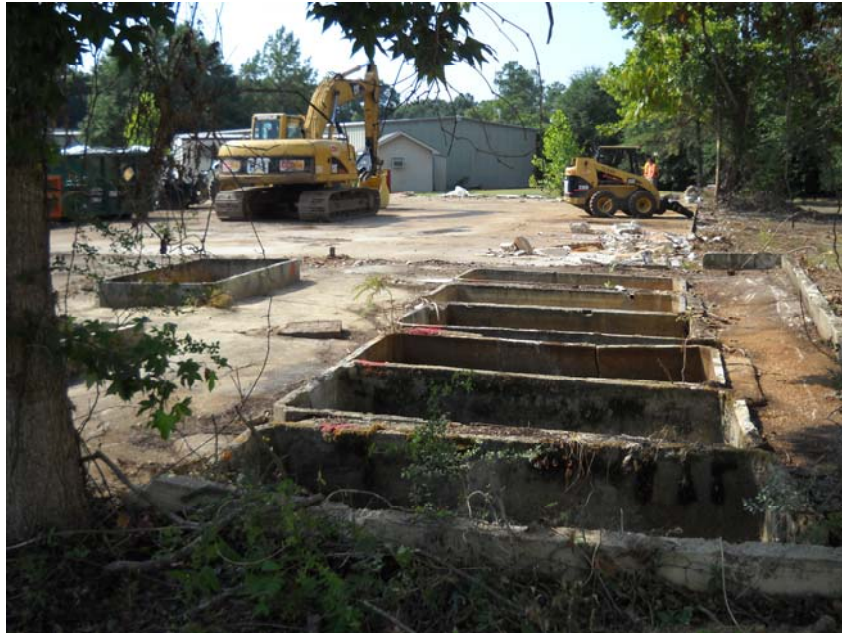
EPA removal of building, concrete pad, and treatment pits
