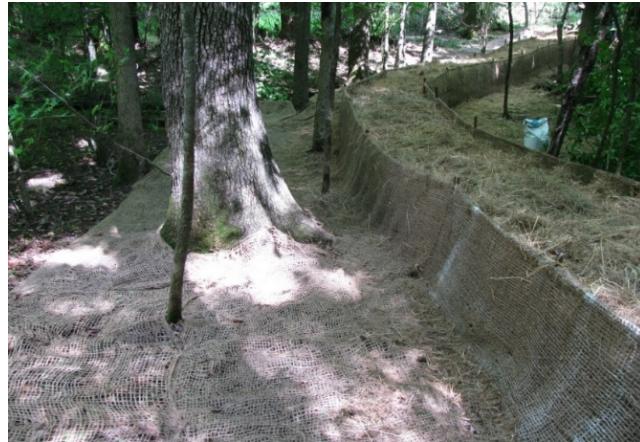
Figure SB-1 Sediment Retention Barrier
