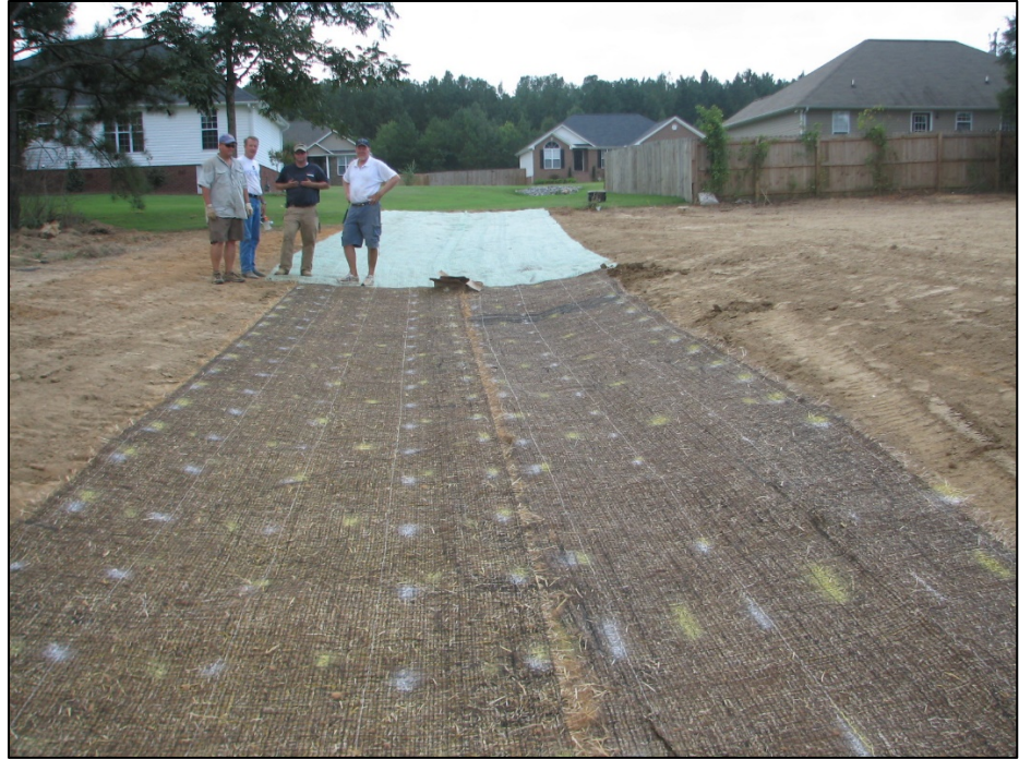
Figure ECB-4 TRM with Pre-Marked Stapling Pattern.
