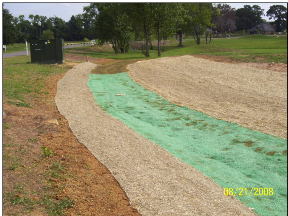
Figure ECB-3 TRM in the Middle of a Swale.
