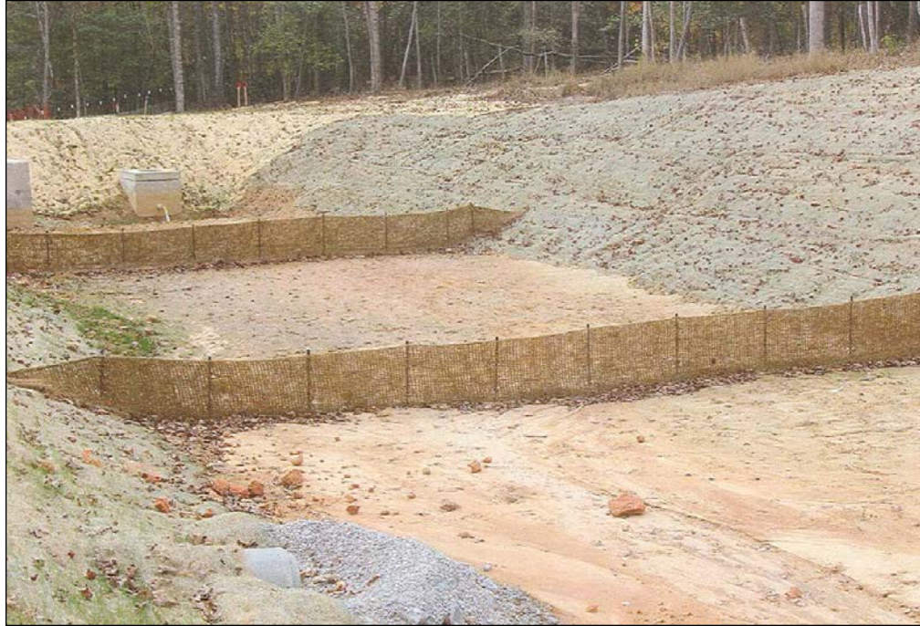
Figure SBN-2 Example of porous baffle made of 700 g/m 2 coir erosion blanket as viewed from the inlet.
