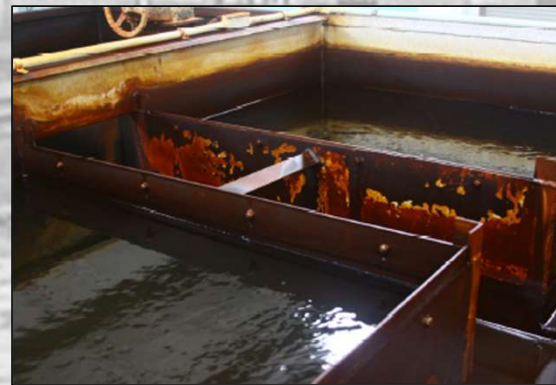
Iron Buildup on the surface of Millport's water treatment unit
