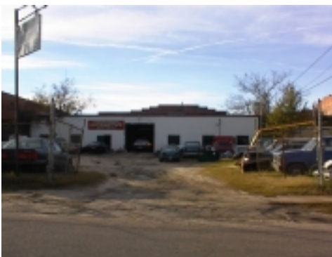
Auto Service Businesses Can Generate Significant Levels of Pollutants If Housekeeping Is Poor or Absent
