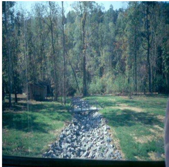
Right: Management measures stabilize this outlet and eliminate future erosion and gully formation from concentrated runoff flow at the Camp.
