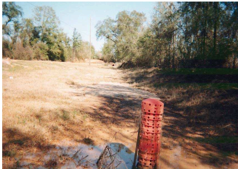
Right: A roadside sediment detention basin at Stephens Ferry Road (Geneva County) helps to protect Sandy Creek, one of the CPYRWMA's first projects to control sediment from unpaved roads.
