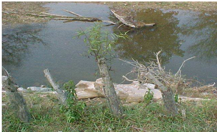
Right: A combination of hard (riprap) and bio-engineered (willow stakes) management measures are used to stabilize a badly eroded shoreline section of Choccolocco Creek.
