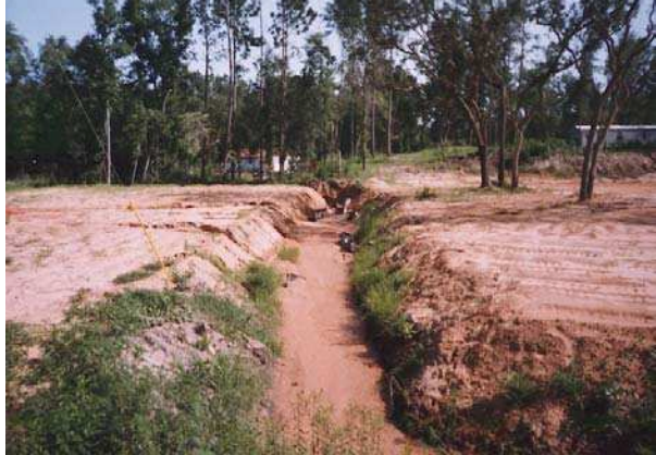
Left and Above: Rapid population growth contributes to a large amount of construction in coastal counties. Land disturbance activities, coupled with some of the highest rainfall intensity in the nation, produces a potential for significant water quality impacts associated with erosion and sedimentation. Several erosion and sediment control workshops have been provided by the Weeks Bay Watershed Project.
