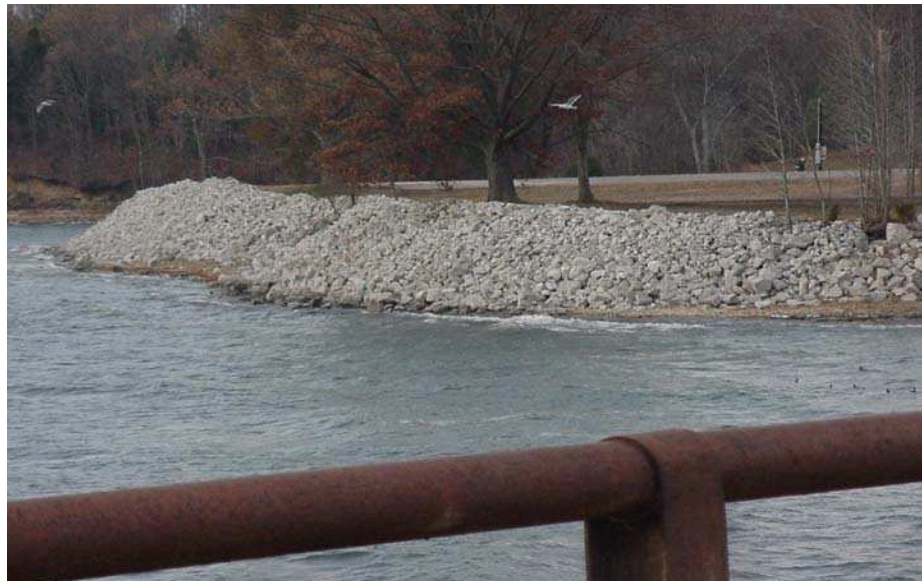
Right: Shoreline after stabilization with sloping and riprap.
