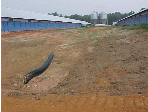
Above: Stabilized outfalls to prevent erosion from runoff are installed on a Barbour County poultry farm as part of the Upper Choctawhatchee Watershed Project.
