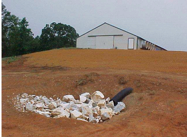
Above: Stabilized outfalls to prevent erosion from runoff are installed on a Barbour County poultry farm as part of the Upper Choctawhatchee Watershed Project.
