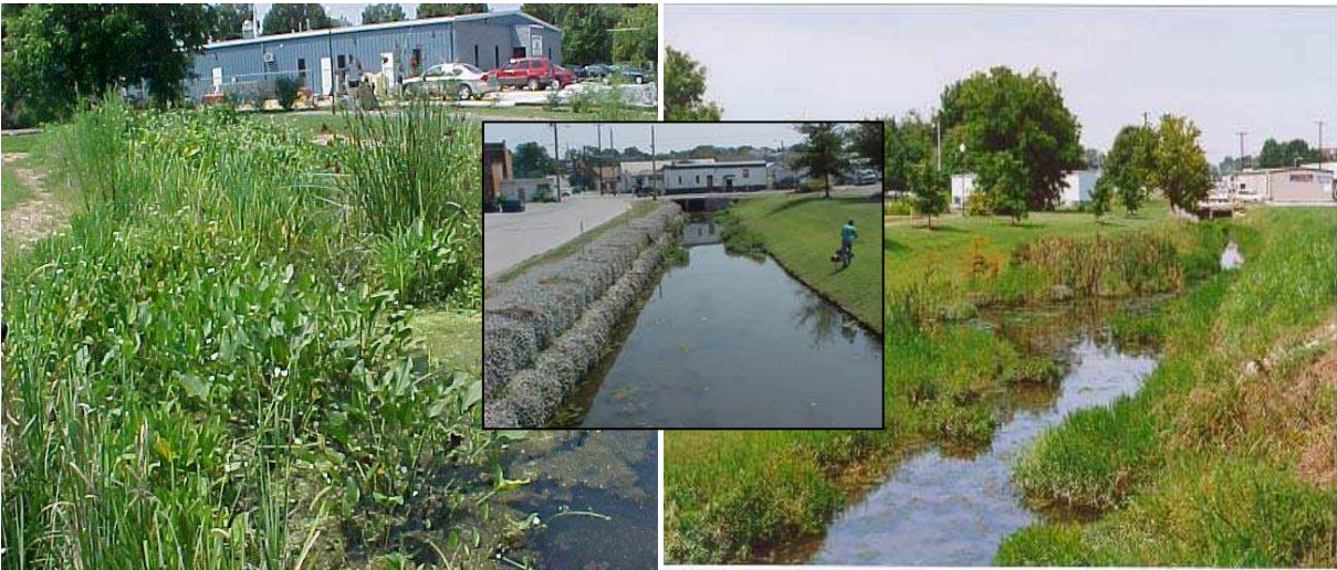
Above, left: After restoration. Middle: Gabion baskets solve undercutting problem (left bank); sloped and grassed (right bank). Above, right: Constructed Wetlands
