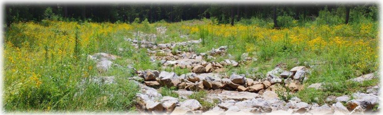
Figure 6: Step pool conveyance system in Joes Branch. Photo Courtesy of Thompson Engineering
