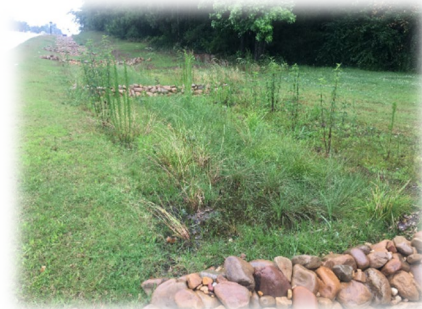
Figure 95: Completed bioswale implemented as part of the project.
