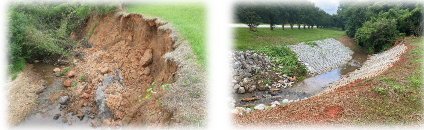
Figure 19: Before (left) and after (right) pictures of the slope stabilization on the tributary to Moores Creek.
