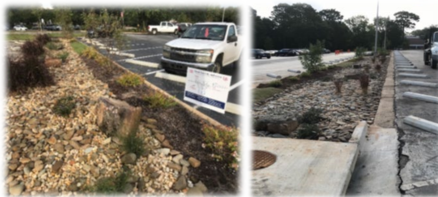
Figure 24: The completed installation of bio-infiltration swales in the USA parking lots.
