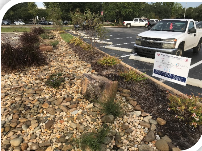
These are the locations for BMP practices for the placements of the bio-infiltration swales in the Humanities Parking lot (above), and a picture of the completed swales (on the right and below).
