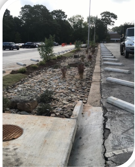
These are the locations for BMP practices for the placements of the bio-infiltration swales in the Humanities Parking lot (above), and a picture of the completed swales (on the right and below).
