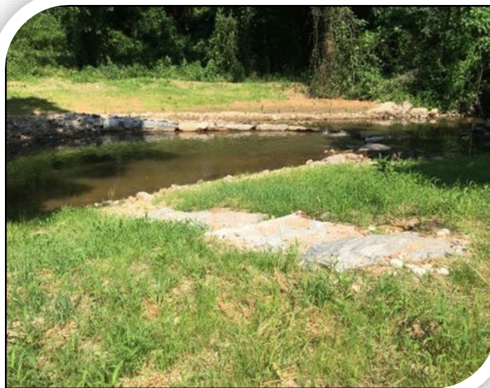
This boulder cross vane redirects the flow of water to the middle of the stream channel, reducing stream bank erosion and adding oxygen to the stream.
