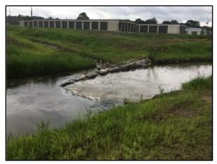
An in-stream stabilization structure was placed to prevent further streambank erosion.
