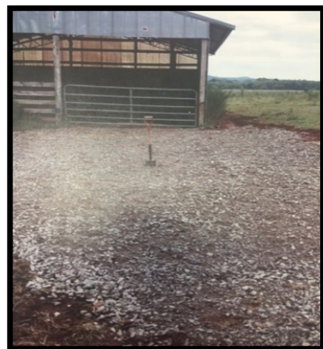
A heavy use area was installed to reduce erosion and nutrients in the Harris Creek Watershed.
