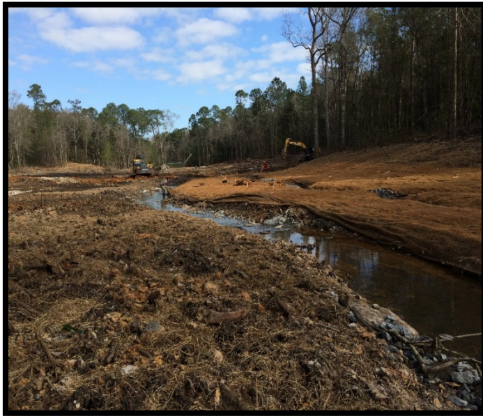
North State Environmental began the stream restoration on the UT to Tiawasee Creek in February 2016.
