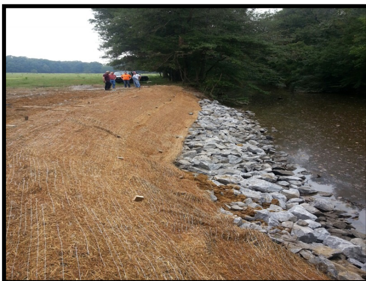
An 85-foot streambank stabilization site was completed on a farm as part of the Broken Arrow Creek Project.
