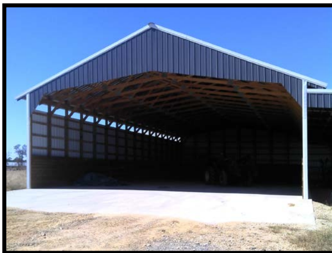
A waste storage structure was constructed to address issues with poultry litter runoff and nutrient management.
