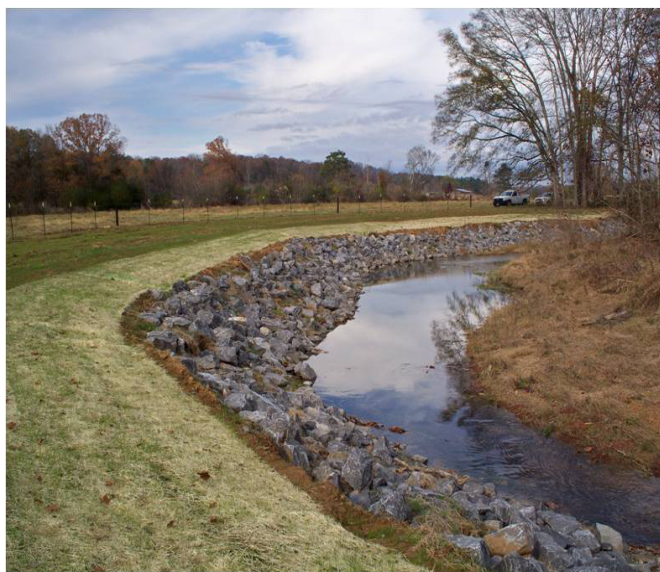
Streambank stabilization on a farm in DeKalb County, before (above) & after (below).
