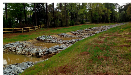
Below: Joe's Branch after the step pool conveyance system was installed
