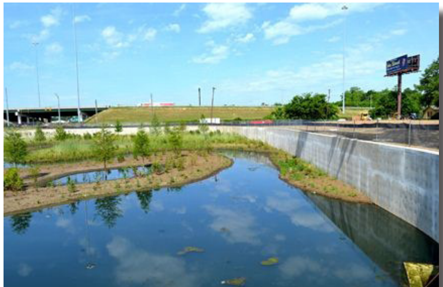
Below: A constructed wetland system has been installed to treat stormwater.
