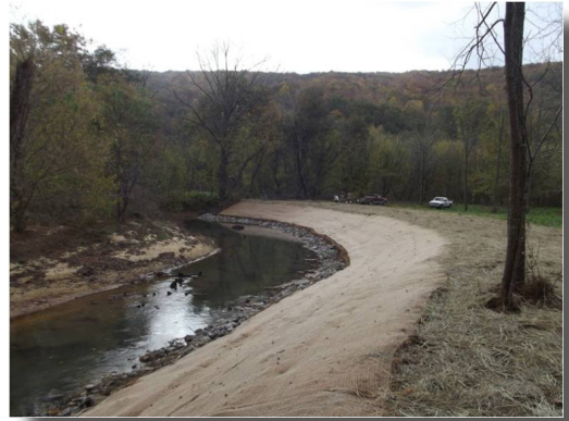
A total of 415 linear feet of streambank was stabilized on two farms.
