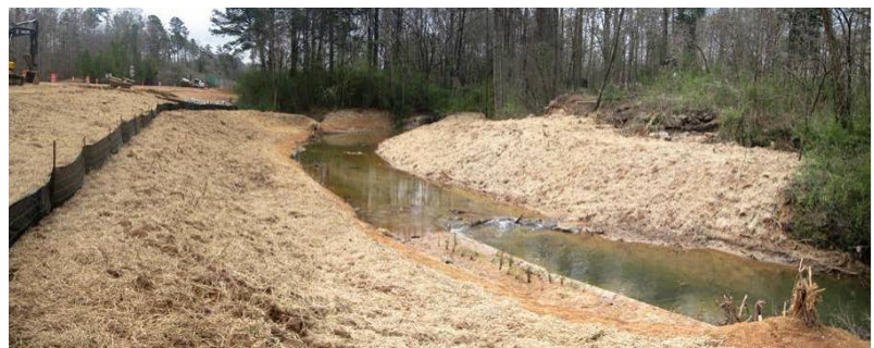
A stream restoration project was completed in conjunction with the City of Auburn's Northeast Sanitary Sewer Project.
