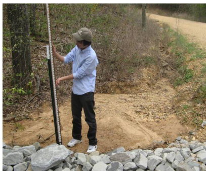
Measuring sediment pollutant loading into an installed detention basin.
