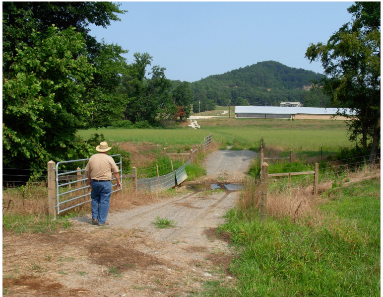
A stream crossing and exclusion fencing for cattle were installed as part of the Dry Creek Project.
