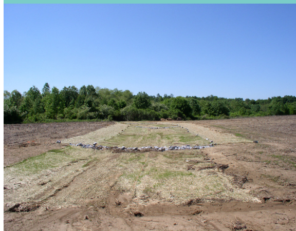
Right and below: A grassed waterway installation, before and after.
