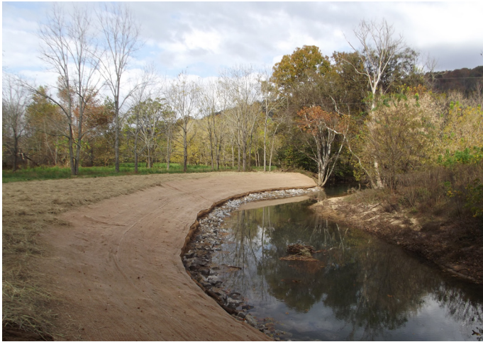
Approximately 140 linear feet of streambank was stabilized as part of the Guess Creek Project.
