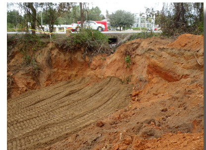
Excavation of the severely eroded stream bed began in October.
