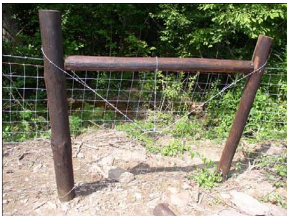
Exclusion fencing for cattle was installed to protect a tributary to Wolf Creek.
