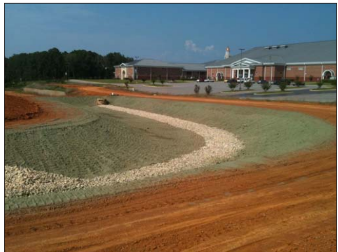
The City of Calera Sports Complex incorporated three bioswales into their existing plans in order to capture runoff.
