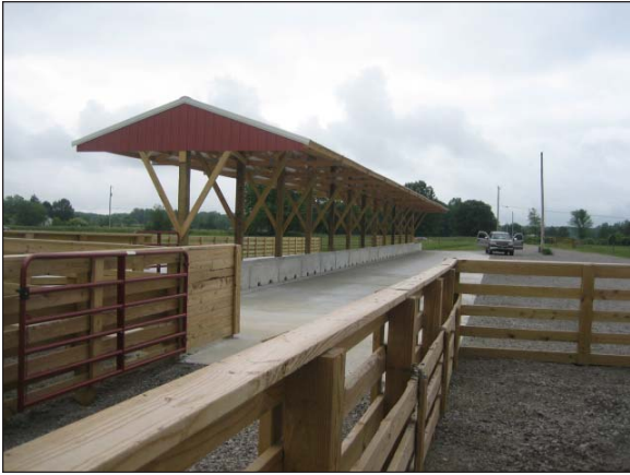
A heavy use cattle feeding area was installed to reduce runoff.
