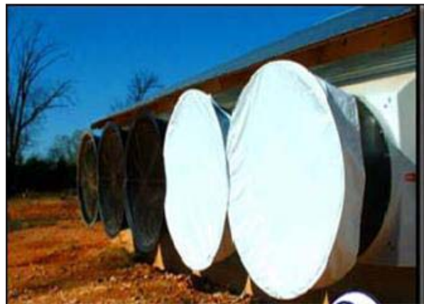
Fan bonnets were installed on fans not being used during cold weather in order to preserve energy.
