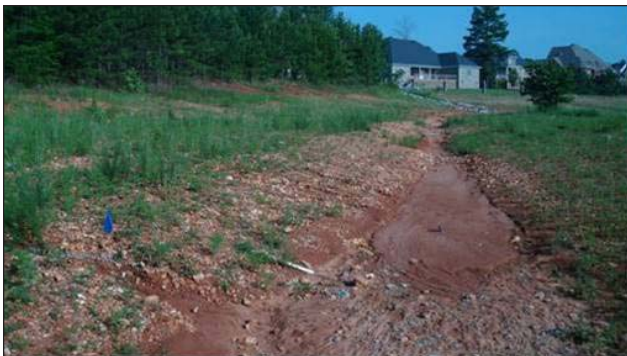
Sparkman High School site before stabilization.
