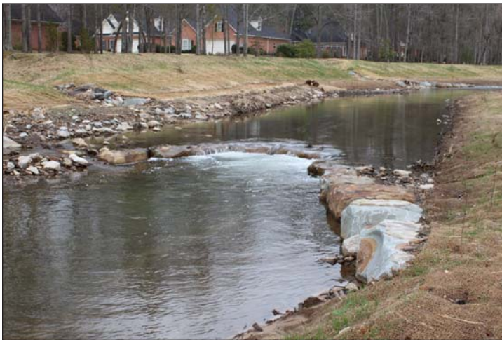
Cross vanes were installed to redirect flow away from streambanks.
