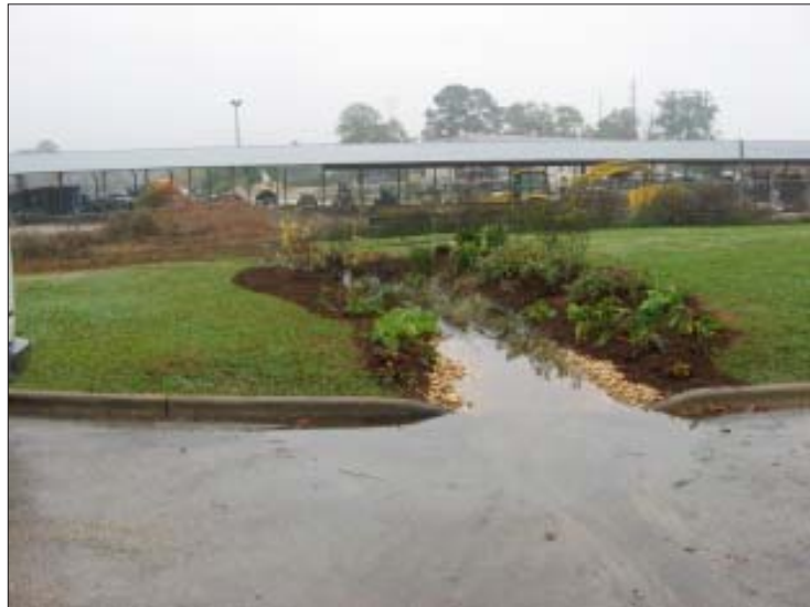
Rain Garden and curbcut to alleviate flooding and catch paking lot runoff at the Boykin Community Center in Auburn.
