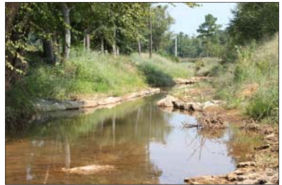
Rock vanes and switch grass were installed as part of the stabilization techniques on Moore's Mill Creek.
