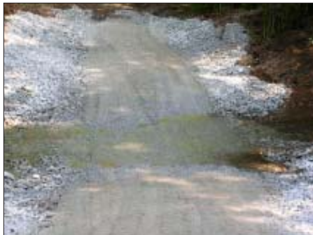
A stream crossing was installed on Wolf Creek for equipment and cattle.
