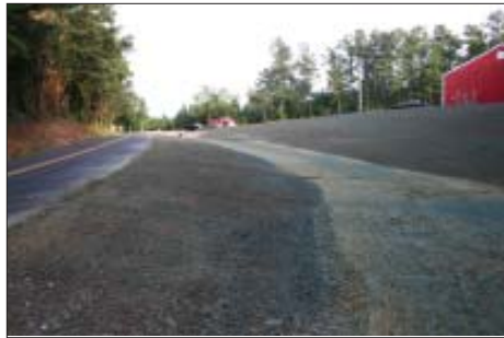
Erosion control blankets and hydroseeding prevent sedimentation.
