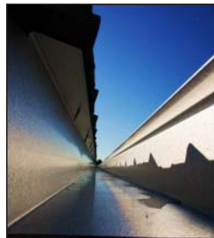
A gutter system installed on a poultry house in the Tennessee Basin.
