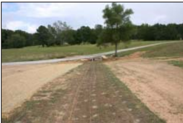
Gully was filled and reshaped prior to hydroseeding and installation of erosion control blankets.
