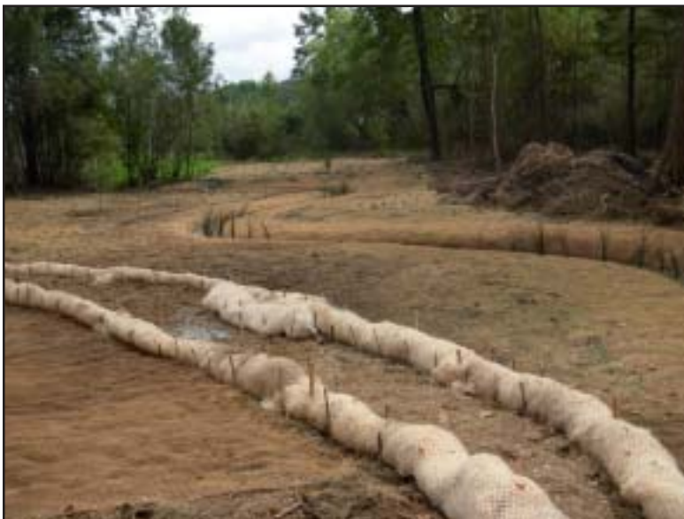
Stream restoration of the Unnamed Tributary nears completion.
