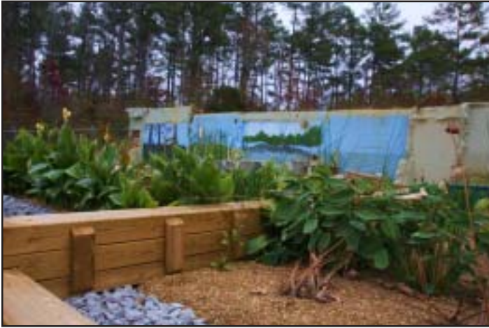
Outdoor wetland cells help treat stormwater runoff in the WaterWorks project.
