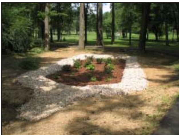
A bioretention area in Ragland treats stormwater runoff from adjacent parking lot.
