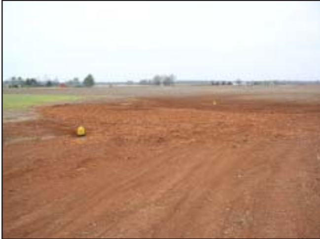
A gully is corrected with a series of sediment basins and an underground outlet.
