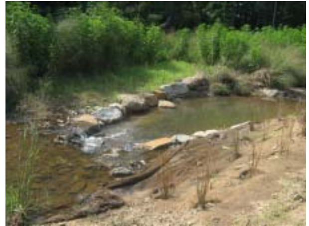
A cross-vane has been implemented as part of the stabilization techniques.
