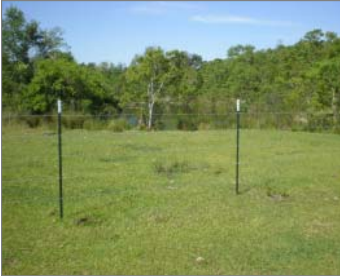
Exclusion fencing along Dowling Branch
