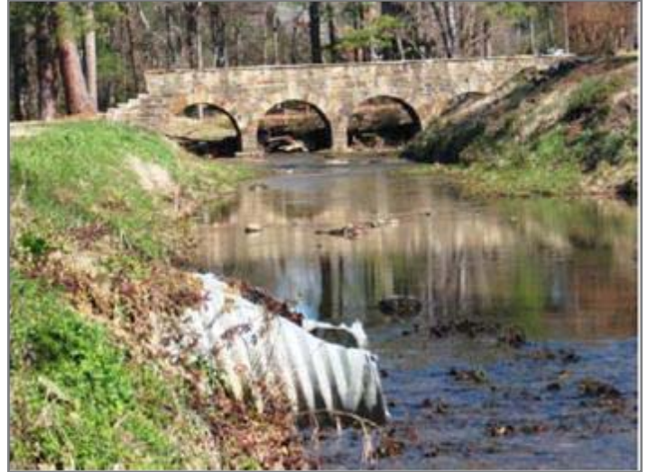
Town Creek prior to construction activities
