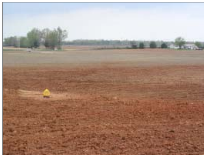
Newly installed sediment basin in the Brier Fork Watershed
