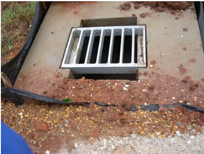
- A Newly installed Stormdrain (Credit: City of Montgomery)
