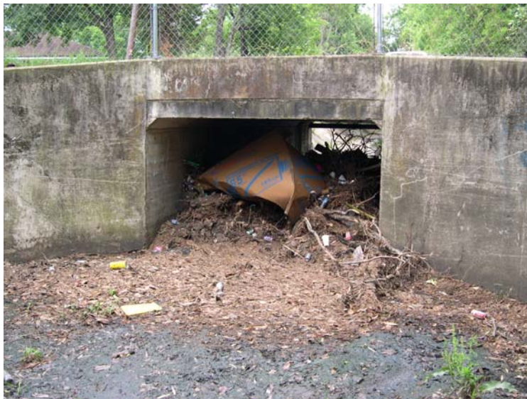
- A Block Culvert near Montgomery (Credit: City of Montgomery)
