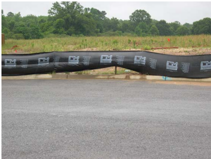
- A Silt Fence (Soil Erosion BMP) at a Road Construction Site near Montgomery (Credit: City of Montgomery)
