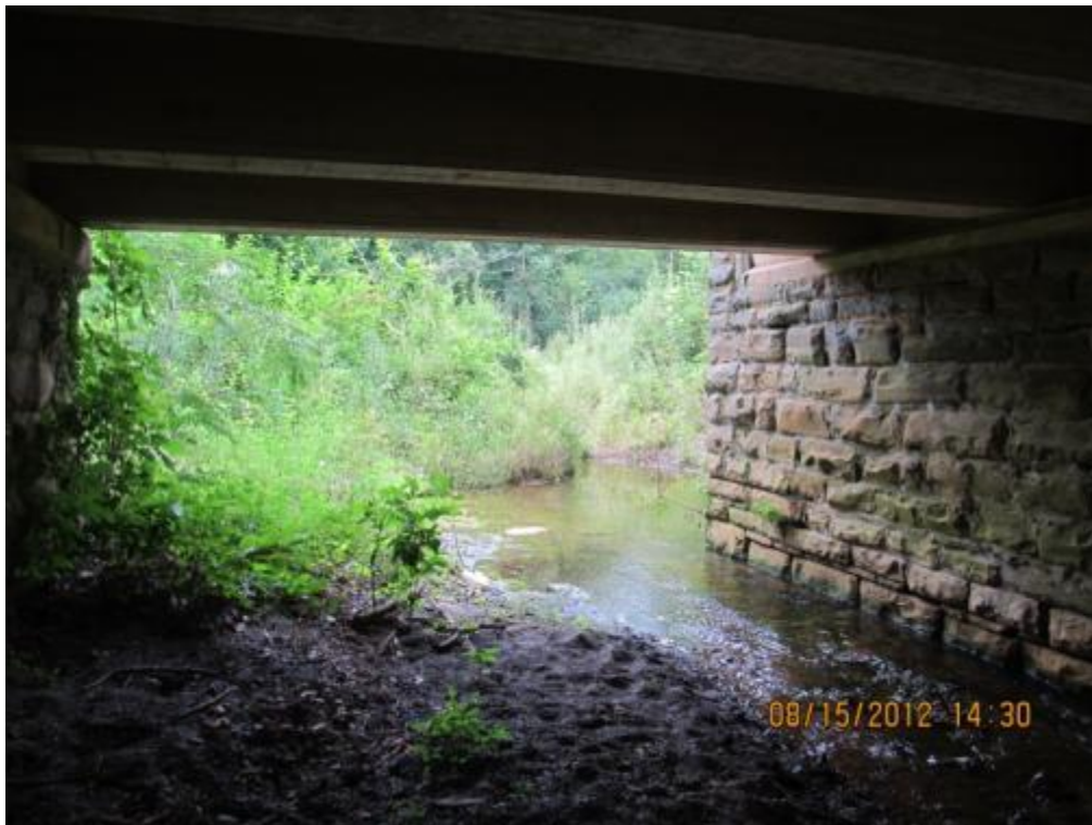
Photo 4 – BKBW-1 Looking Downstream (Photo Taken 8/15/2012)
