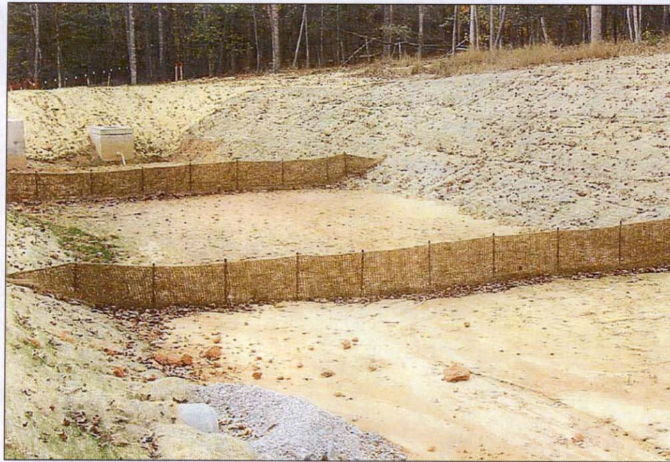
Figure SBN-2 Example of porous baffle made of 700 g/m 2 coir erosion blanket as viewed from the inlet. (from North Carolina Erosion and Sediment Control Planning and Design Manual.)
